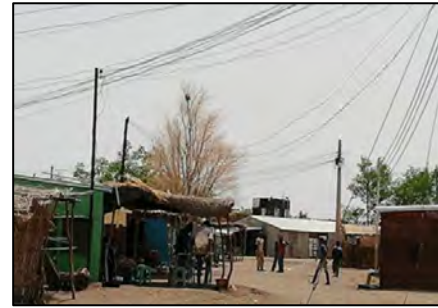
Photo 6 - Electricity available in the market area only
