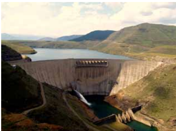
Figure 1: LHWP: Katse Dam
